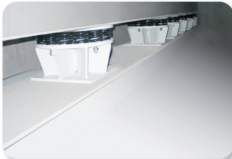
Vibration isolation of a foundation with steel spring isolators SSI-D with integrated damping
